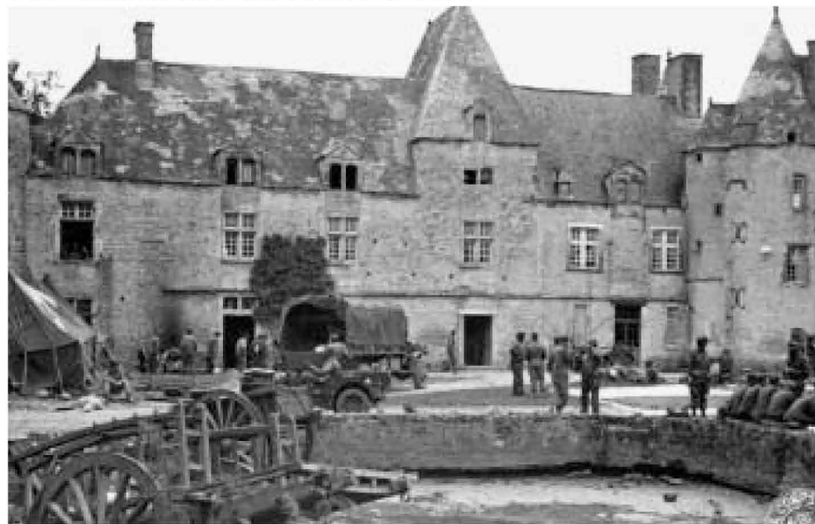
On June 9, 1944, at 11:35 pm, two German bombs scored direct hits on the Château de Colombière at Hiesville. The chateau housed a medical facility where many casualties of the 101st Airborne Division were being treated at the time.
